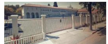
An example of a new fence
